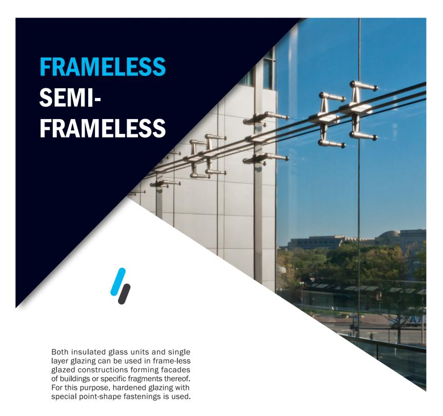
Glazing with point-shape fastenings with the help of special details – "spiders" is fastened to columns, building roofing's, walls or specially equipped metal structures. Seams between the glasses are filled with special sealant.
