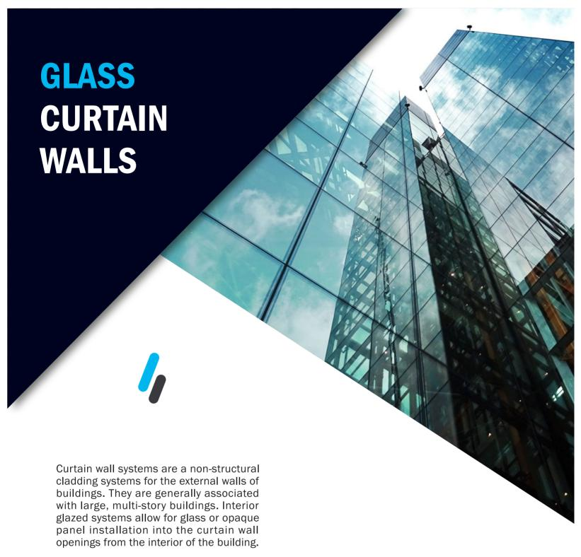
Exterior glazing systems work well for low rise construction projects that allow for easy access to the exterior of the building. Larger high-rise construction projects may require interior glazing.
